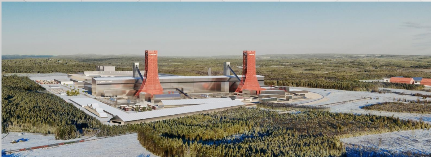
H 2 Green Steel Electric Arc Furnace with H 2 DRI feeding
